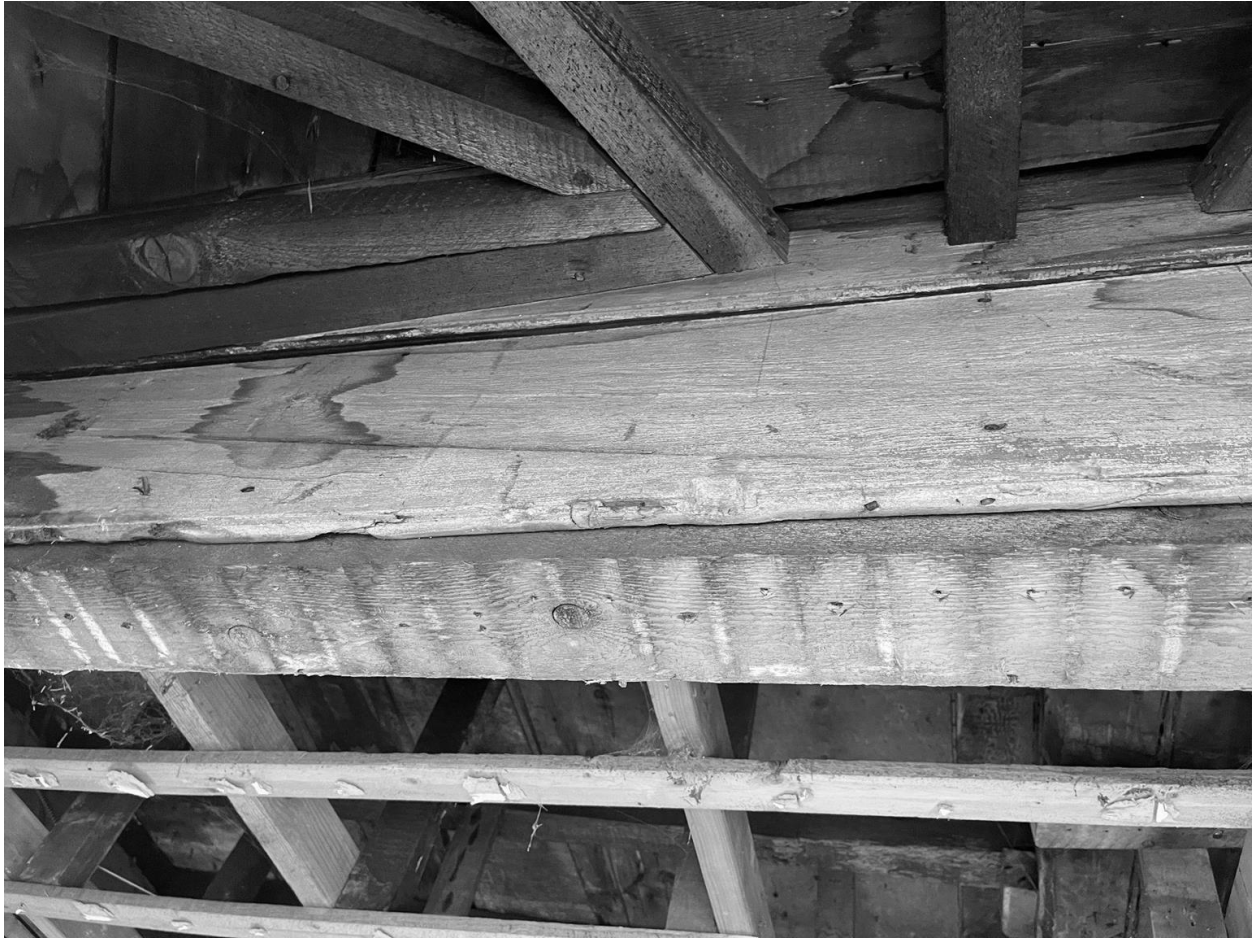
Photo 14. First Story SW Room - Early exterior siding at South Wall
