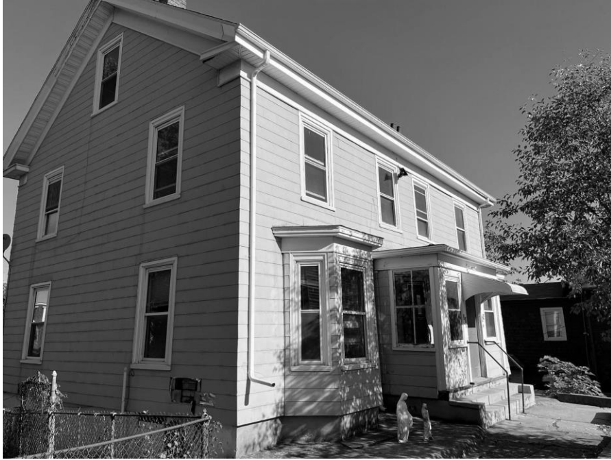
Photo 5. West elevation and south facade
