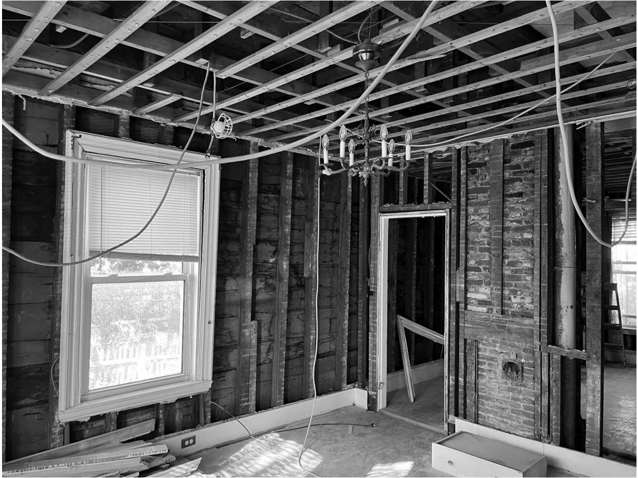
Photo 13. First Story SW Room - West & North Walls
