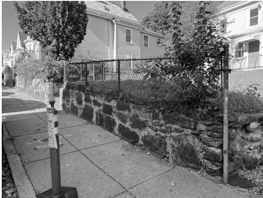
Photo 2. South boundary of property showing retaining wall
