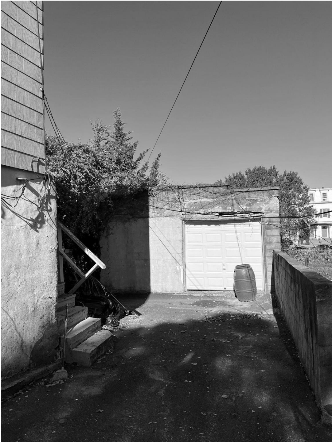
Photo 8. South facade of garage
