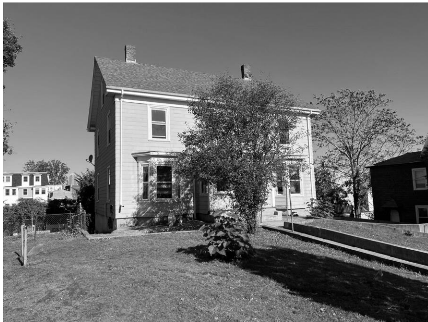
Photo 4. West elevation and south facade
