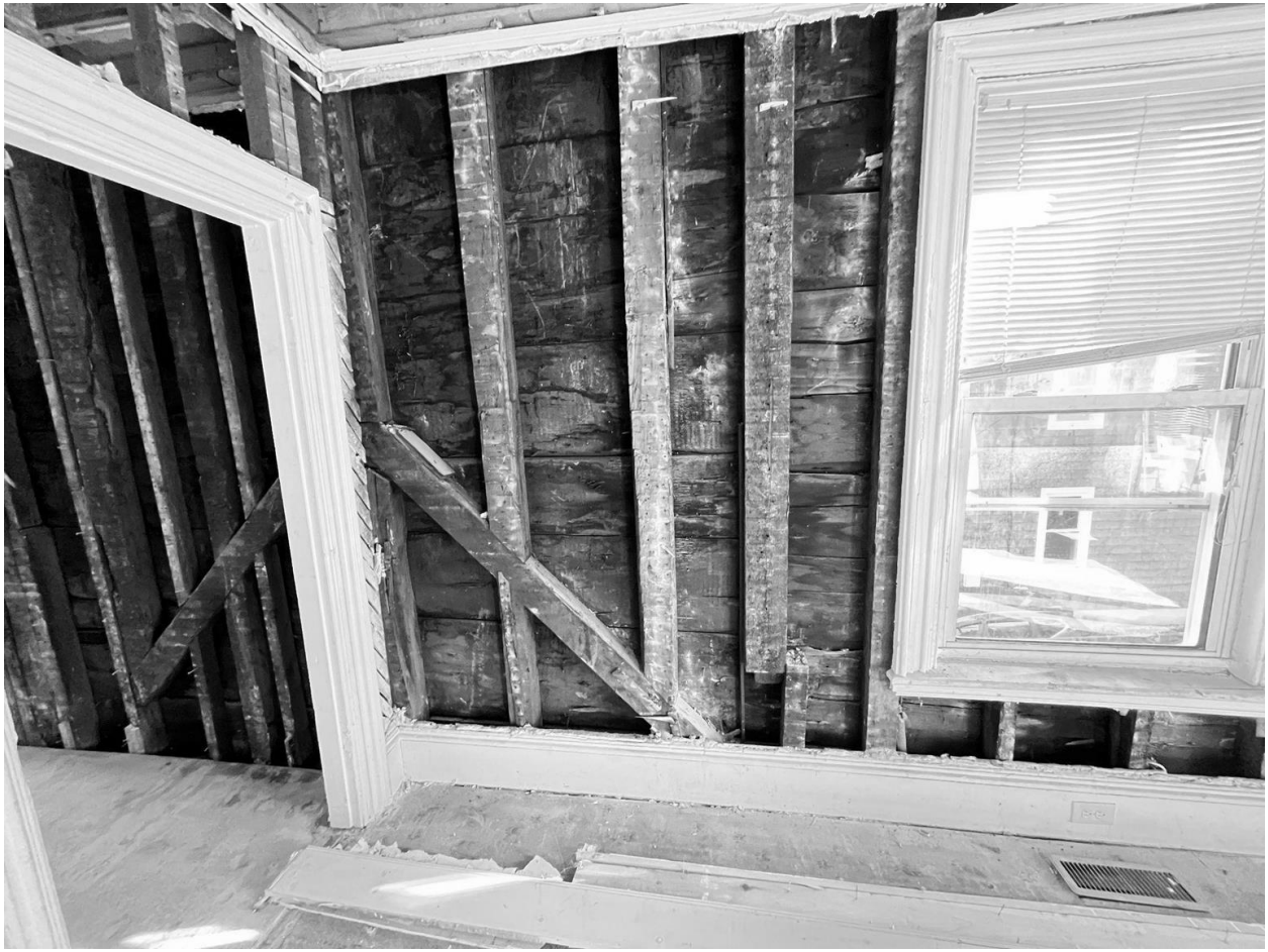
Photo 15. First Story SE Room - North & East Walls
