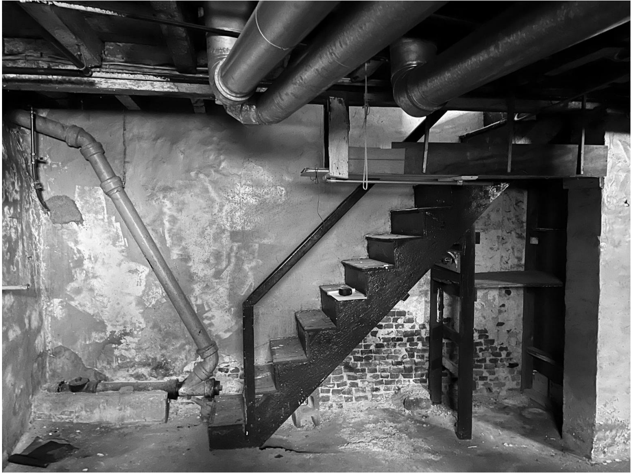
Photo 17. Basement, SE Room - West Wall
