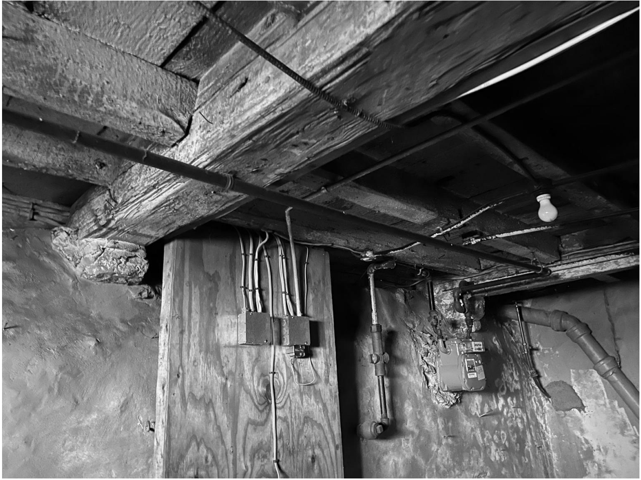
Photo 18. Basement, SE Room - Detail of historic framing
