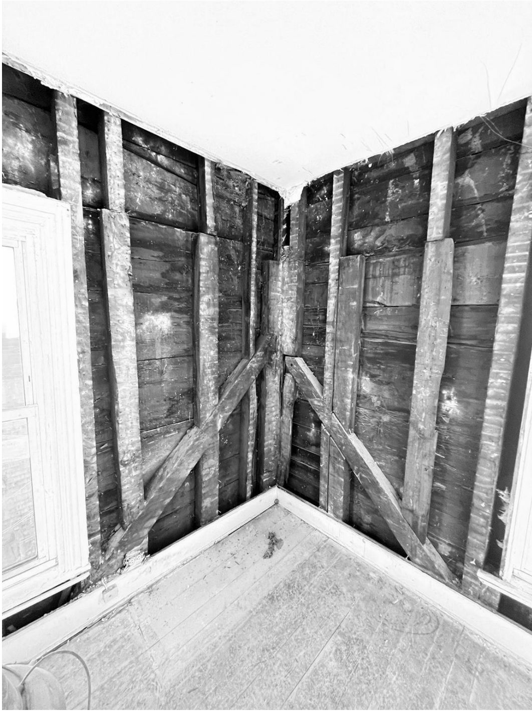
Photo 16. Second Story NE Room - North & East Walls
